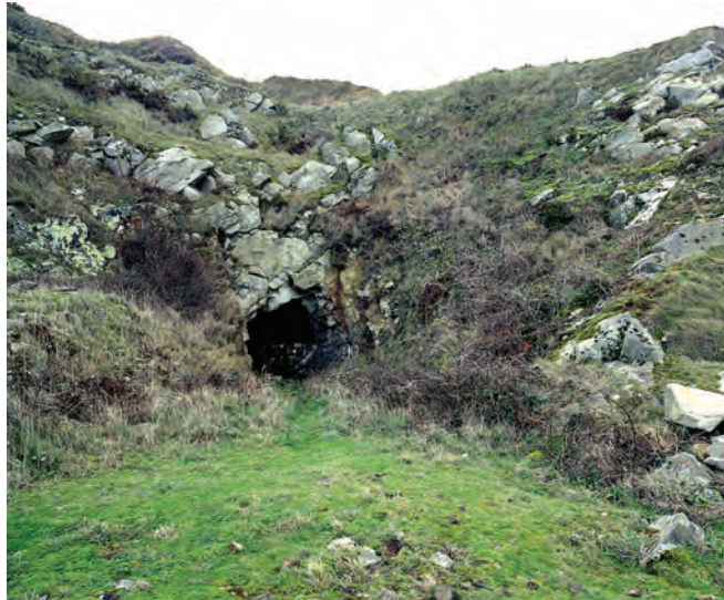
Entrance to Ho 1 in Mannez Quarry. The unlined tunnel is cut through sandstone and consists of a loop with two entrances, 142 metres in length. It was used to store munitions and rations.
